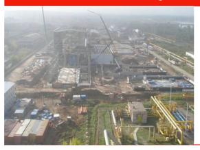
Foundation works completed; Start of installation of metal structures framework
